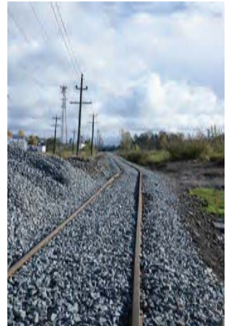
By-pass track is laid on top of the sub-base, ballast is applied. Above, the old line is left, centre is for grain cars, right is new bypass. Below the new FVHRS track passes the culvert and drain seen in previous photos. Below right, the old line is now cut at the Red flag.
