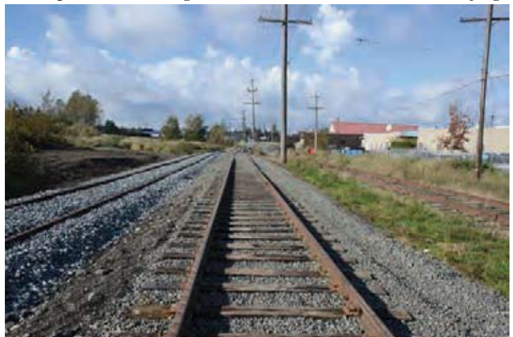
By-pass track is laid on top of the sub-base, ballast is applied. Above, the old line is left, centre is for grain cars, right is new bypass. Below the new FVHRS track passes the culvert and drain seen in previous photos. Below right, the old line is now cut at the Red flag.
