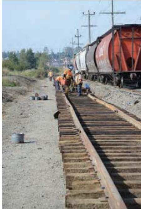
By-pass track is laid on top of the sub-base, ballast is applied. Above, the old line is left, centre is for grain cars, right is new bypass. Below the new FVHRS track passes the culvert and drain seen in previous photos. Below right, the old line is now cut at the Red flag.
