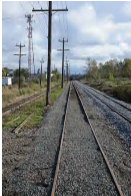
By-pass track is laid on top of the sub-base, ballast is applied. Above, the old line is left, centre is for grain cars, right is new bypass. Below the new FVHRS track passes the culvert and drain seen in previous photos. Below right, the old line is now cut at the Red flag.
