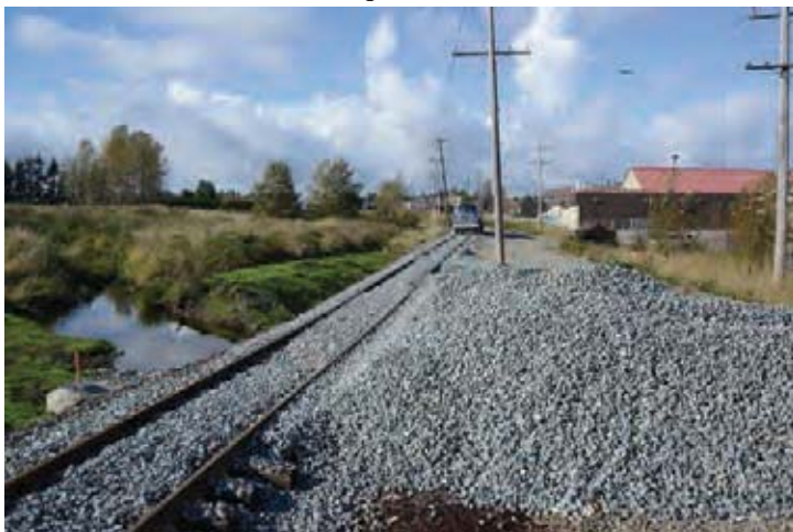
By-pass track is laid on top of the sub-base, ballast is applied. Above, the old line is left, centre is for grain cars, right is new bypass. Below the new FVHRS track passes the culvert and drain seen in previous photos. Below right, the old line is now cut at the Red flag.
