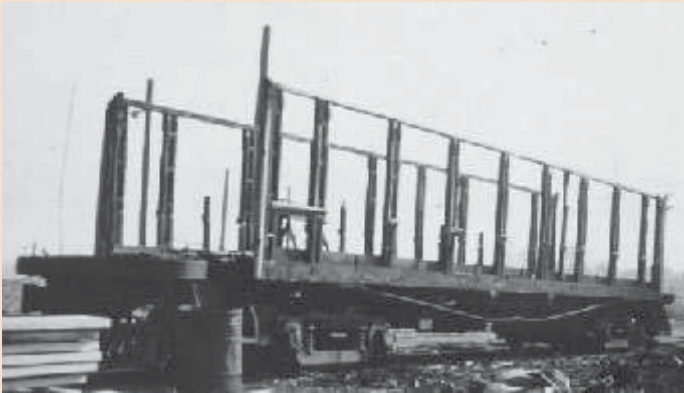
Left: 1304 chassis, after all the burned materials were removed in preparation for rebuilding. (Right) 1304 leading a Chilliwack train, newly-rebuilt following the devastating fire.
