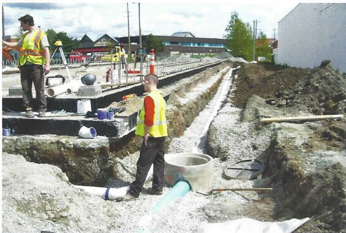
End of April installing the perimeter drains
