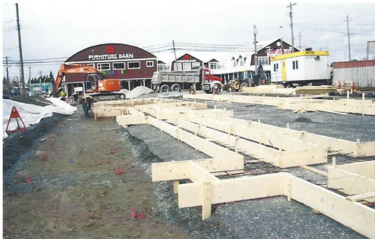
Cloverdale site construction pics March 20 - 31 1212: Foundations for the Car Barn.
