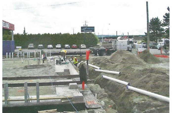
End of April installing the perimeter drains
