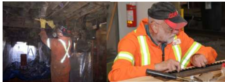
Scraping the underside of the car Rene Doyharcabal fitting woodwork
